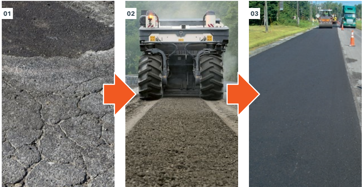
01 - 04 In cold recycling, damaged asphalt layer are granulated, mixed with binding agents, processed, compacted, and repaved.
