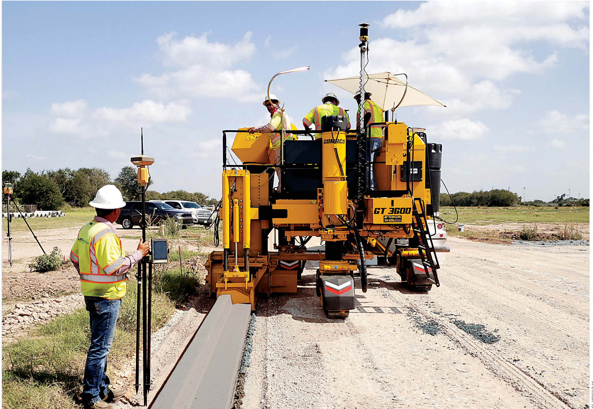
An 18 inch (457 mm) curb and gutter is slipformed using 3D machine guidance by the Xtracore GT-3600 in a new residential development.
