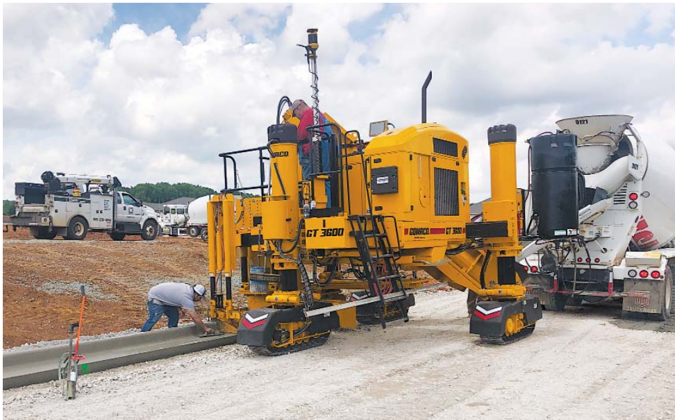
A GOMACO Xtreme GT-3600 slipforms curb and gutter for a new subdivision using 3D machine guidance.
