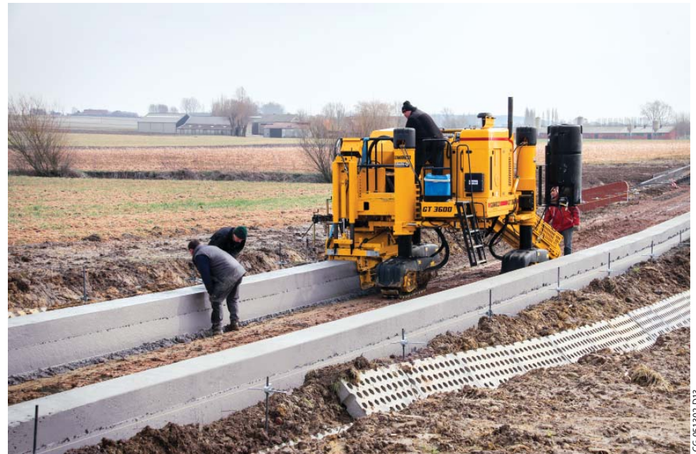
A flood defense barrier is being slipformed by the GT-3600 for a small village in Belgium.
