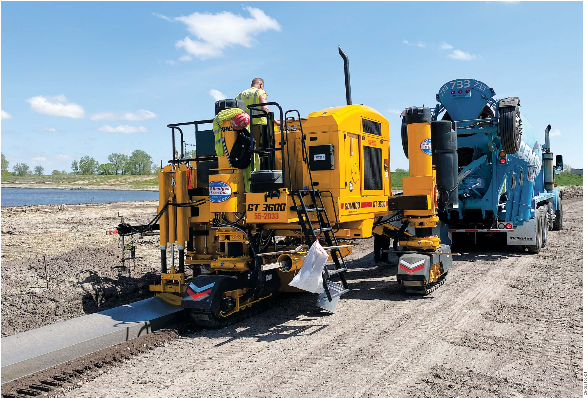
The Xtreme GT-3600 slipforms roll-over curb in a new developmental area.
