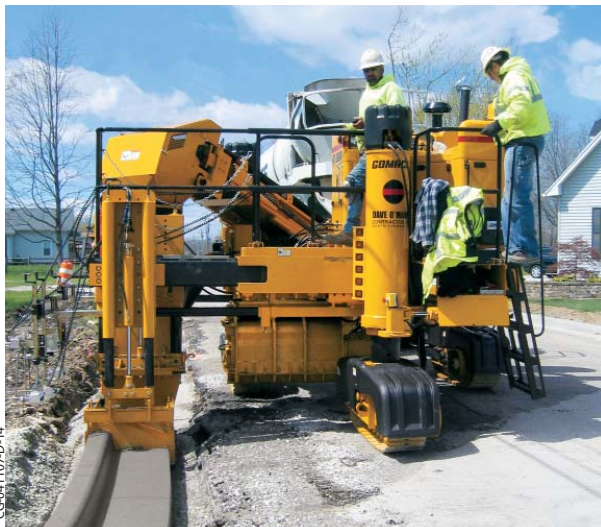
Tight-clearance paving is accomplished with the sideshifting capability of the mold.
