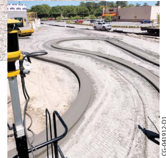
Parking lot island radii are a breeze with the Xtreme GT-3600's steering capabilities and 3D machine guidance. Combining the sensed All-Track Steering and sensed All-Track Positioning has made the Xtreme GT-3600 the ultimate, intelligent slipform curb and gutter machine.
