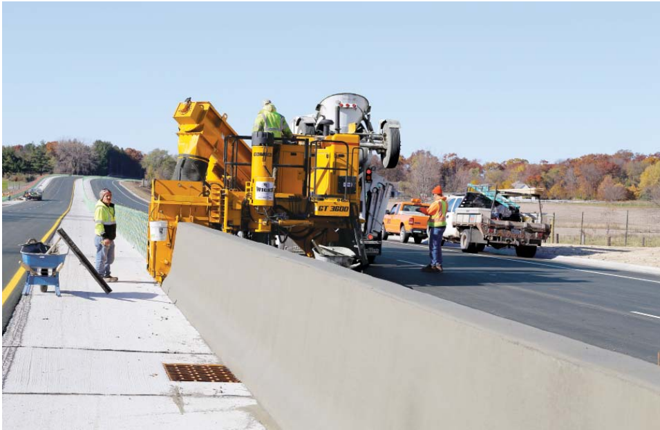
GOMACO's GT-3600 slipforms a 44 inch (1118 mm) median barrier.
