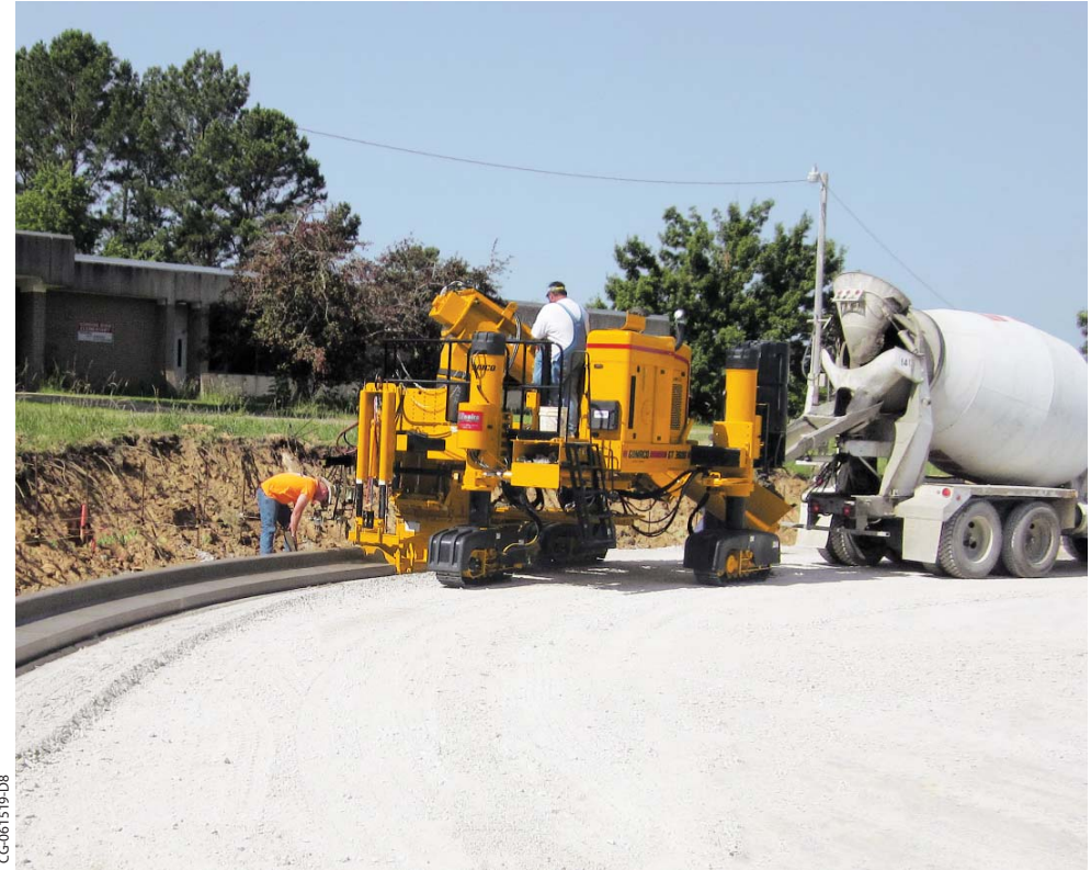
The GT-3600 slipforms curb and gutter around a cul-de-sac in a new residential development.
