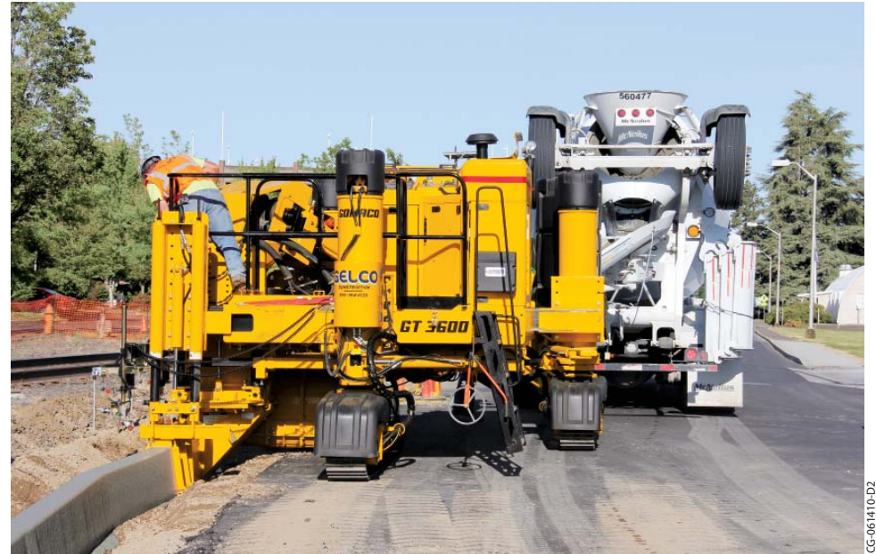
The GT-3600 slipforms stand-up curb.
