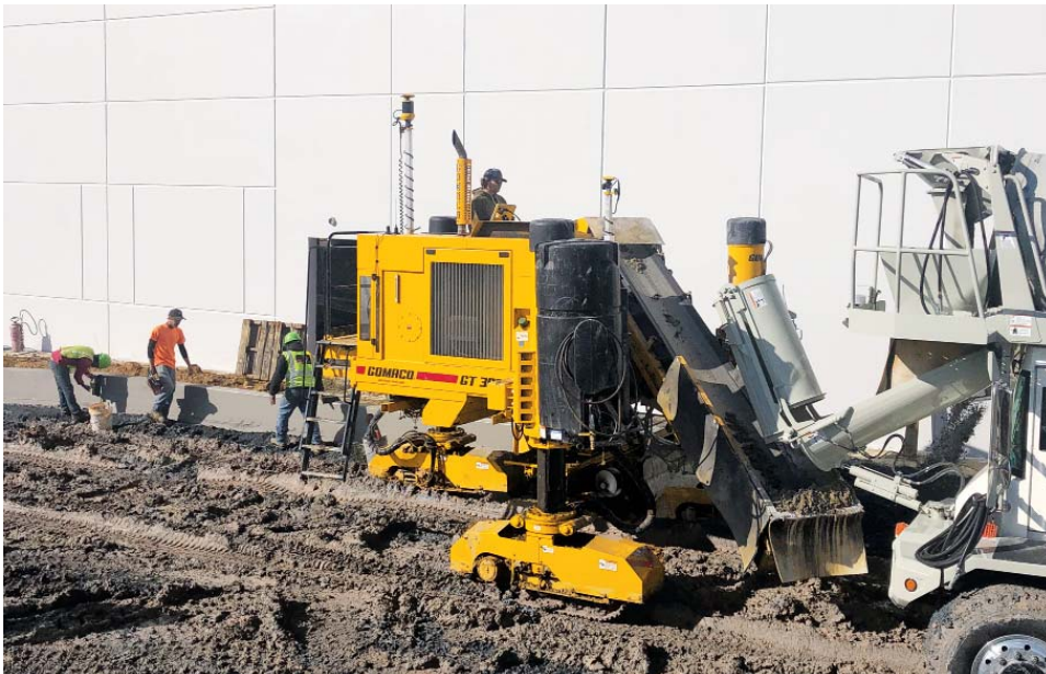
The 16 foot (4.88 m) long conveyor aids the Xtreme GT-3600 as it slipforms 21 inch (533 mm) tall stand-up curb by feeding the hopper at a maximum belt speed of 284 feet per minute (86.6 mpm).
