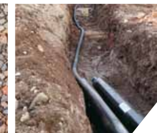
Reused for backfilling
