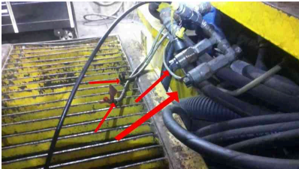
Brake sensors broken, need to be replace
