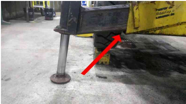
Right outrigger loose,tefflons haves to be replace
