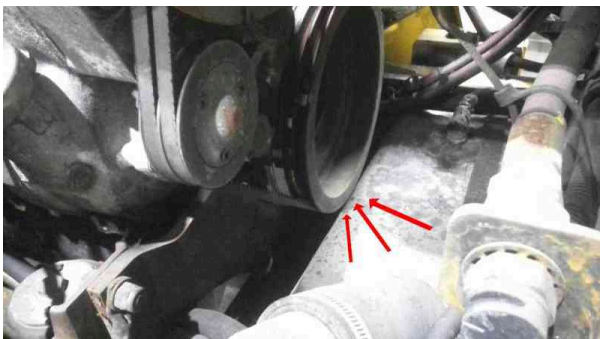
Fuel tank strap is not attach to the brackets and tank is damage by the engine damper pulley
